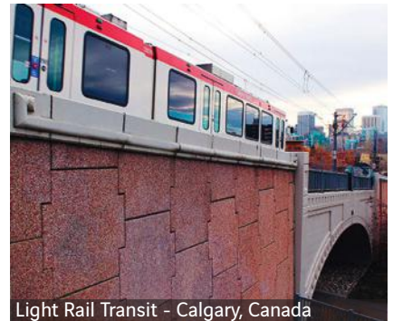
Light Rail Transit - Calgary, Canada
