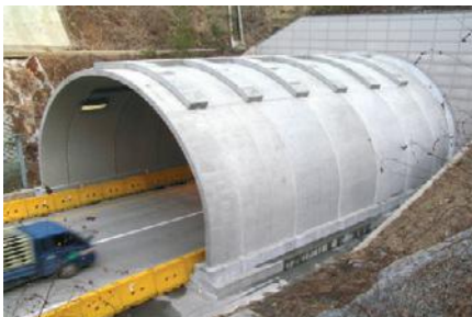
Tunnel extension - Hyeongok (South Korea)
