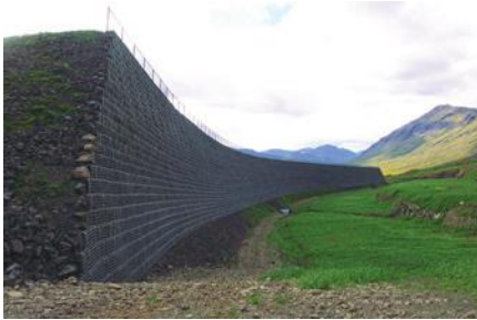
Avalanche barrier - Neskaupstadir (Iceland)
