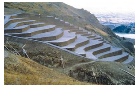
Stabilization of landslide - Caimmuir (New Zealand)
