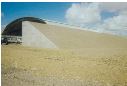
Blast barrier - Townsville (Australia)
