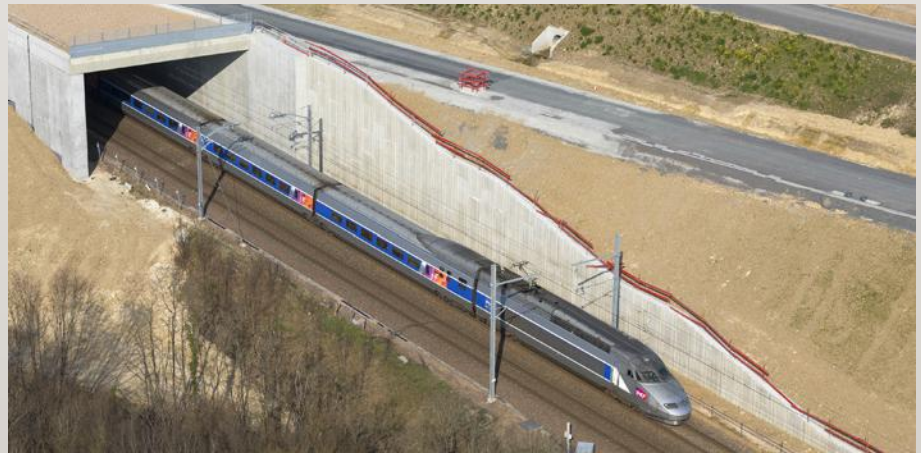
SEA high-speed rail project (France)
