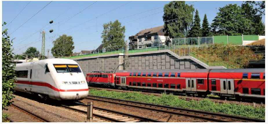
Haan Gruiten (Germany) – Reinforced Earth walls with sound absorbing facing
