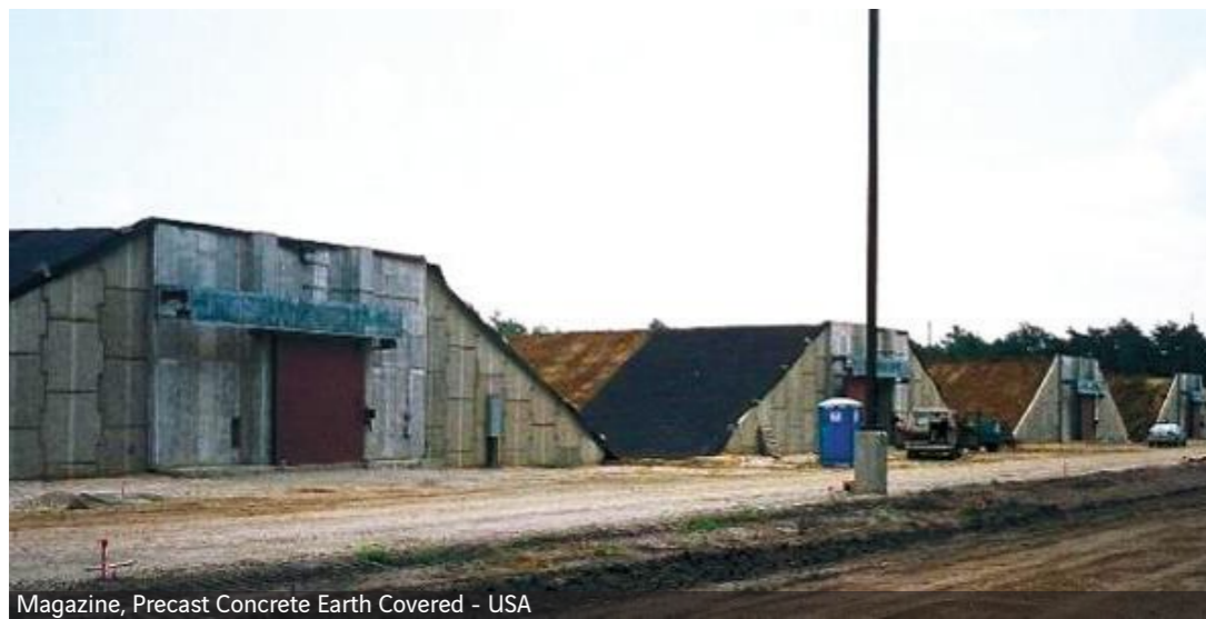
Magazine, Precast Concrete Earth Covered - USA
