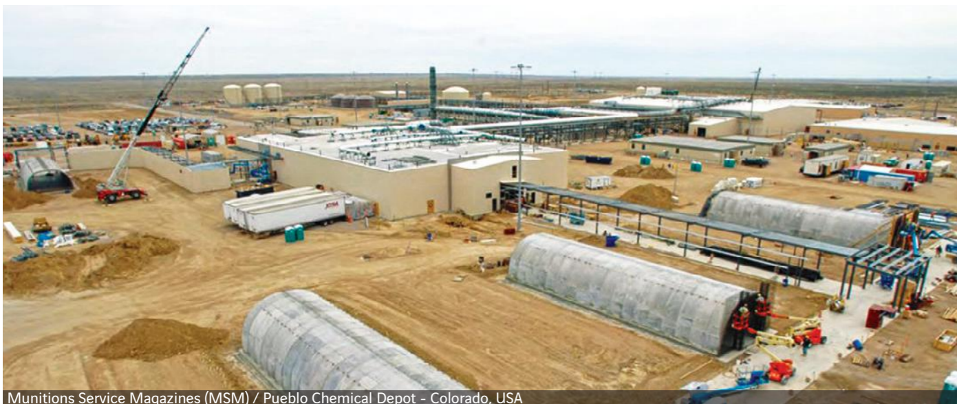
Munitions Service Magazines (MSM) / Pueblo Chemical Depot - Colorado, USA
