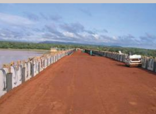
Kromellenboog dam, South Africa
