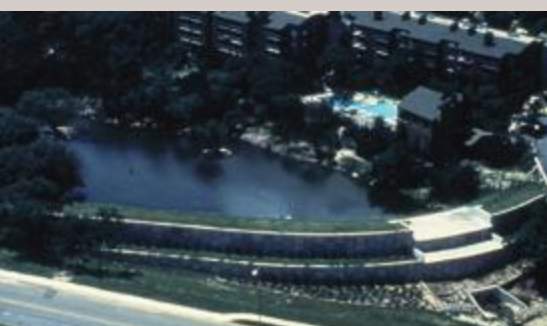
Woodhollow dam, Texas, USA
