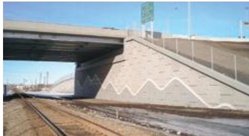
Open abutment with straight wing walls
