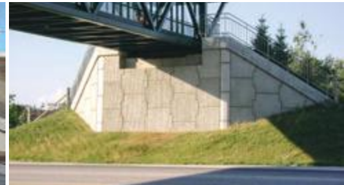
Open abutment with oblique wing walls
