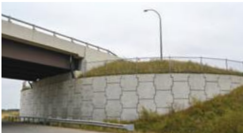
Open abutment with inwardly curved wing wall
